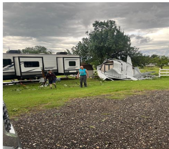
Brent with Dennis who found his storage shed was wrapped by a metal carport that went airborne from 3 lots over.
